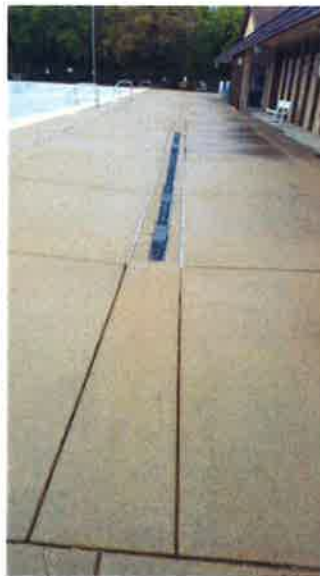
typical trench drain
