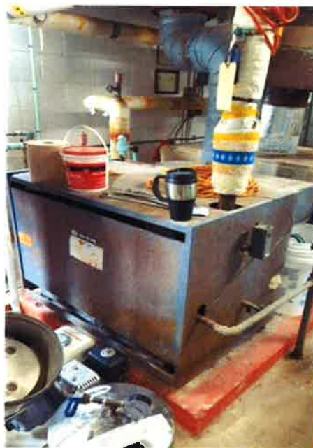
Boiler for radiant floor heat (abandoned)
