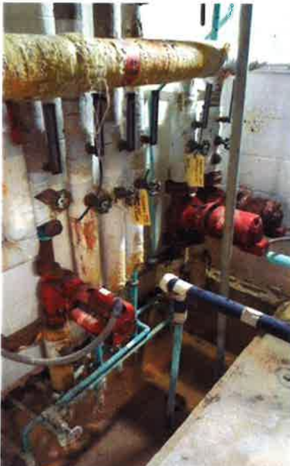
Zone pumps for radiant floor heat
