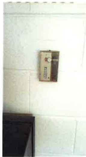
Thermostat for radiant floor heat
