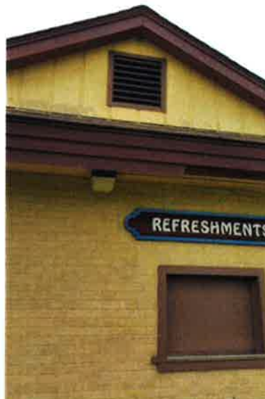
Typical exhaust louver for bathhouse
