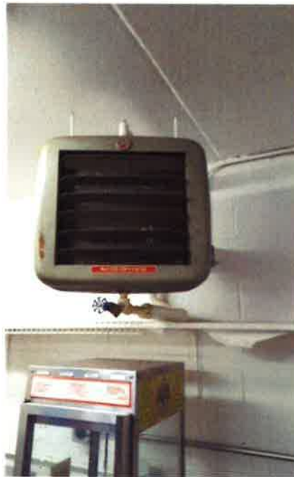
Hot water unit heater in Concessions
