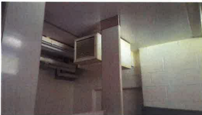
Exposed exhaust ductwork in Bathhouse
