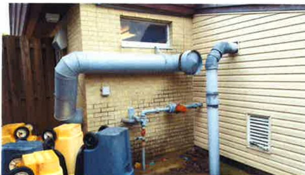
Exterior intake venting for pool heater
