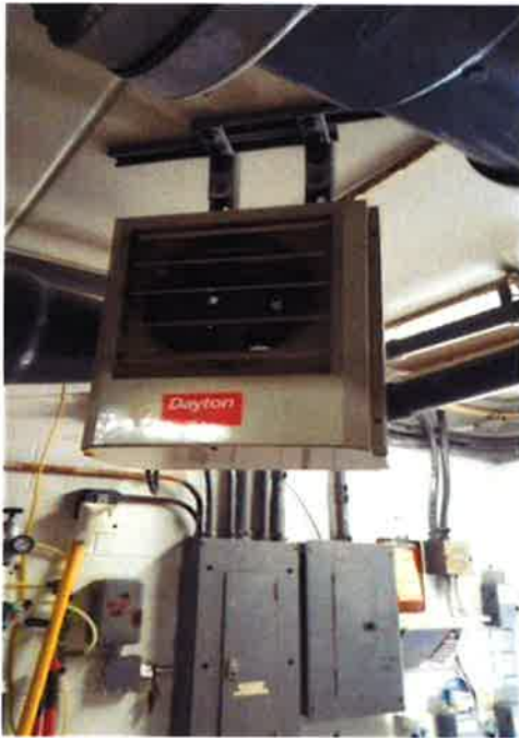
Electric unit heater in boiler room
