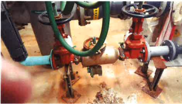
Backflow preventer for pool fill
