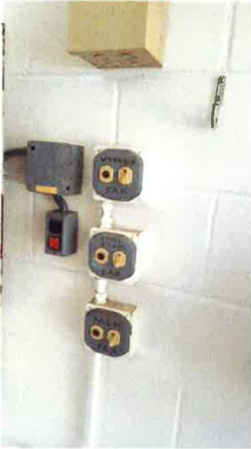
Switches for Bathhouse Exhaust fans
