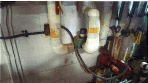
Backflow preventer for pool fill
