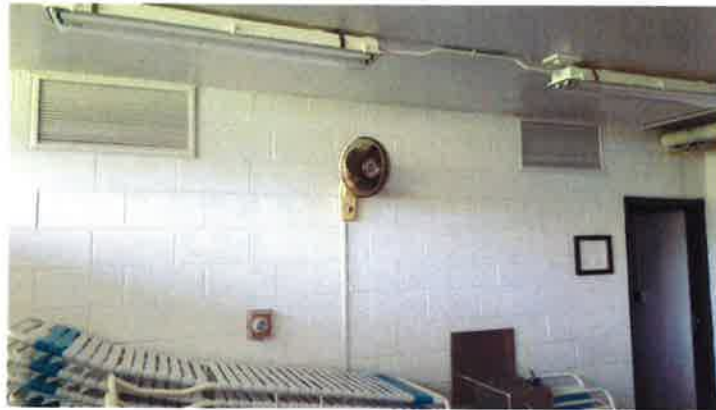
Typical exhaust grilles in Bathhouse
