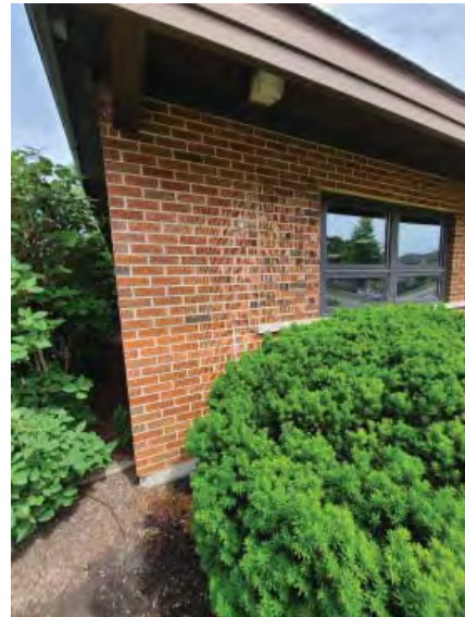
NO GUTTERS, EXISTING WEATHERED FASCIA
