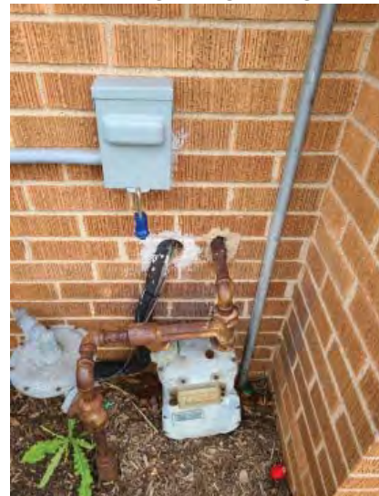
NOT PROPERLY SEALED PENETRATIONS INTO THE BUILDING
