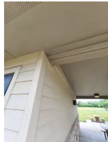
FAILING CAULK
