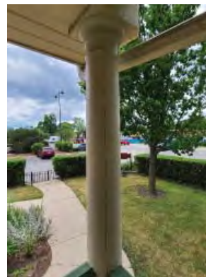
CRACKED COLUMN COVER
