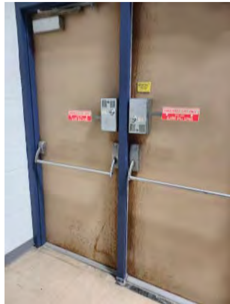
EXISTING DOORS ARE RUSTED
