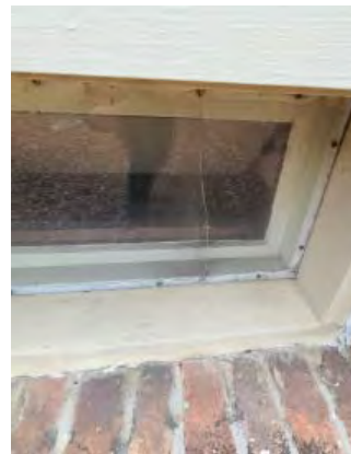
BROKEN BASEMENT WINDOW
