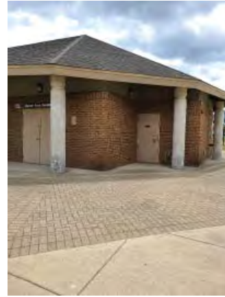
NO GUTTERS, EXISTING WEATHERED FASCIA
