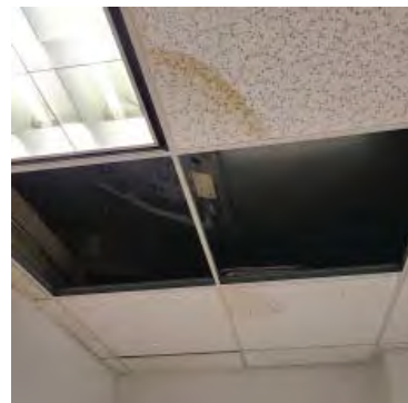
CEILING TILES MOVED, STAINS ON CEILING
