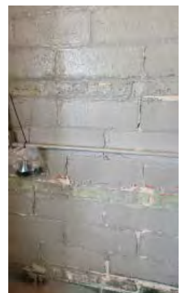
STEP CRACKS IN WALL
