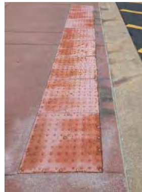
DETECTABLE WARNING FAILING
