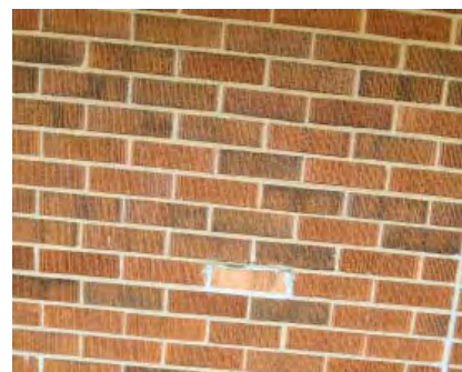
POORLY CAULKED BRICK
