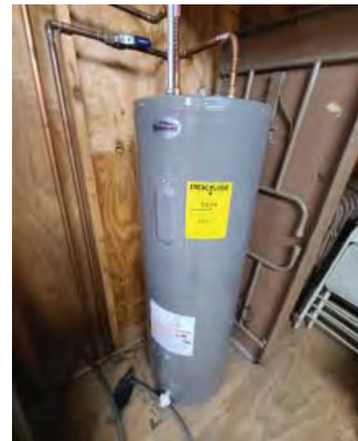
WATER HEATER WITHOUT PAN AND
