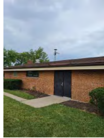
NO DOWNSPOUTS AT THE REAR EXIT DOOR
