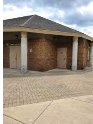
NO GUTTERS, EXISTING WEATHERED FASCIA
