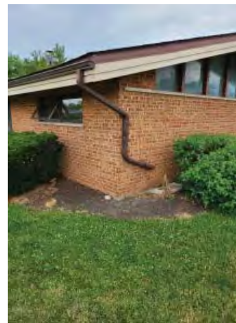
DOWNSPOUT DRAINING AT BUILDING
