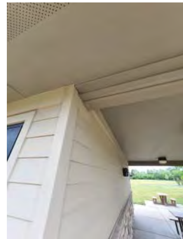
FAILING CAULK
