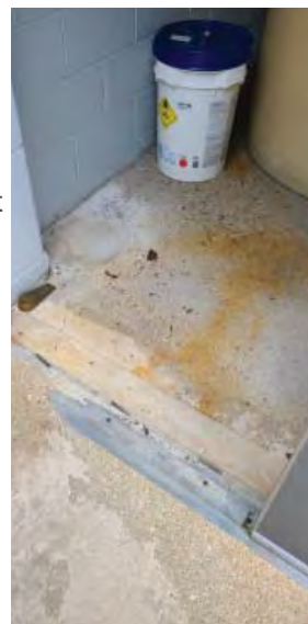
THRESHOLD HAS DETERIORATED
